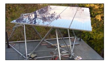
Array in its horizontal position. Picture taken at the end of the installation.
