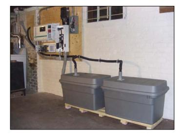
The two large plastic containers house the batteries. The black hose takes the hydrogen from the containers to an unused chimney. The electronics on the wall form the power control center for the house. Picture was taken during the inspection process when all covers were removed from critical components.
