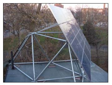
Array tilted at about 65 degrees. Picture shows tilting mechanism. The support structure, designed by Ben Rodgers of Solsmart Energy Solutions Inc., consists of three interlocked tetrahedra. Each strut is 7 feet 6 inches (2.286 m) long consisting of 2.38 inch (6.03 cm) OD schedule 40 steel pipe.
