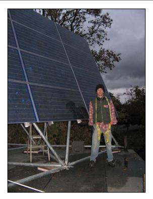
This picture is included to show the actual size of the array with respect to a person. The array is 12 square meters (129.1 square feet) in area. It is shown as the finishing touches were being made to the installation.
