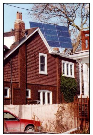
The array as seen from Ravina Crescent. The solar panels are fabricated from a crystalline substrate giving them a mottled blue/indigo appearance in the sunlight. They are manufactured by Centennial Solar Inc. of Montreal.
